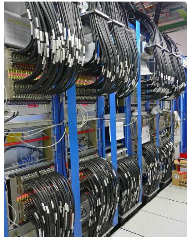
Cabling from Receiver to L1Calo
