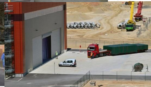
PF conductor arriving ITER site
