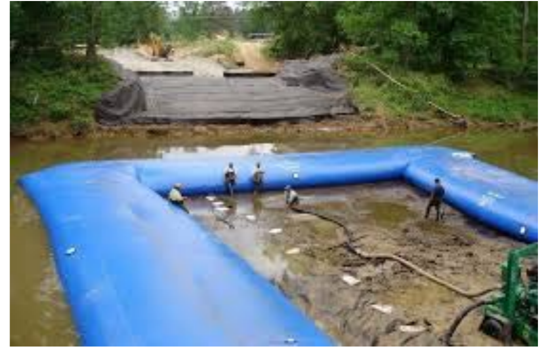
Coffer Dam technology can prepare area for building
