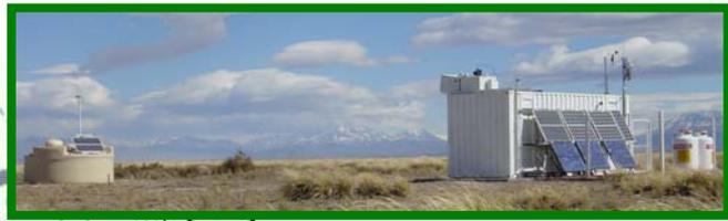
**1600 surface detector stations: water-Cherenkov tanks (triangular grid of 1.5 km)**
