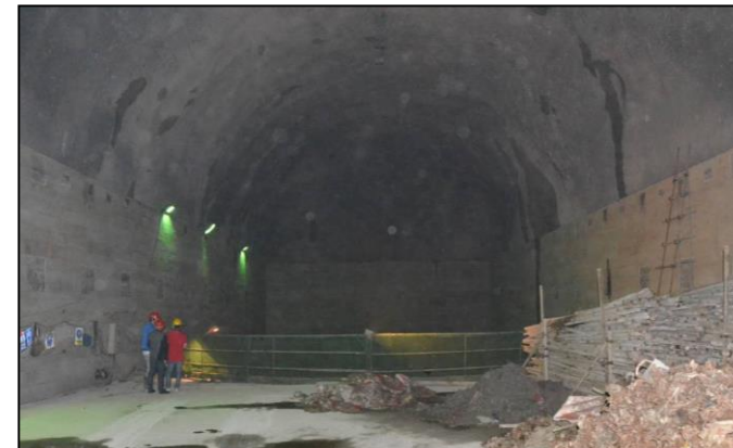
PandaX foundation pits
