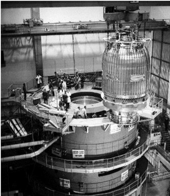
**BEBC project ( 1966) giant cryogenic bubble chamber surrounded by a 3.5 T superconducting solenoid magnet that operated at CERN Super Proton Synchrotron (SPS) until 1984**
