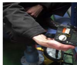
Insulation resistance check
