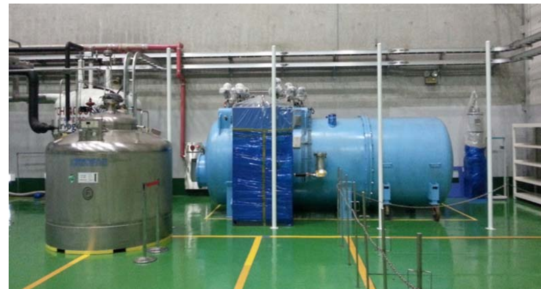
Assembly in the KSTAR building
