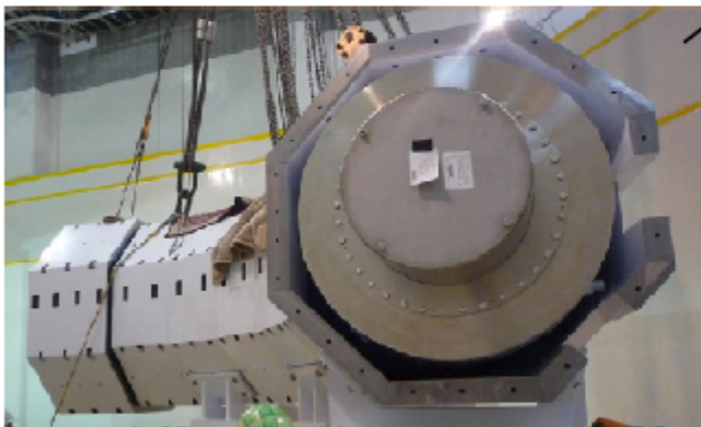
Transport Solenoid Installed
