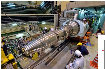
Final focusing SC magnet and cryostat
