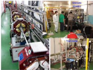
Fig. 4: ILC ATF2 beam line magnets
