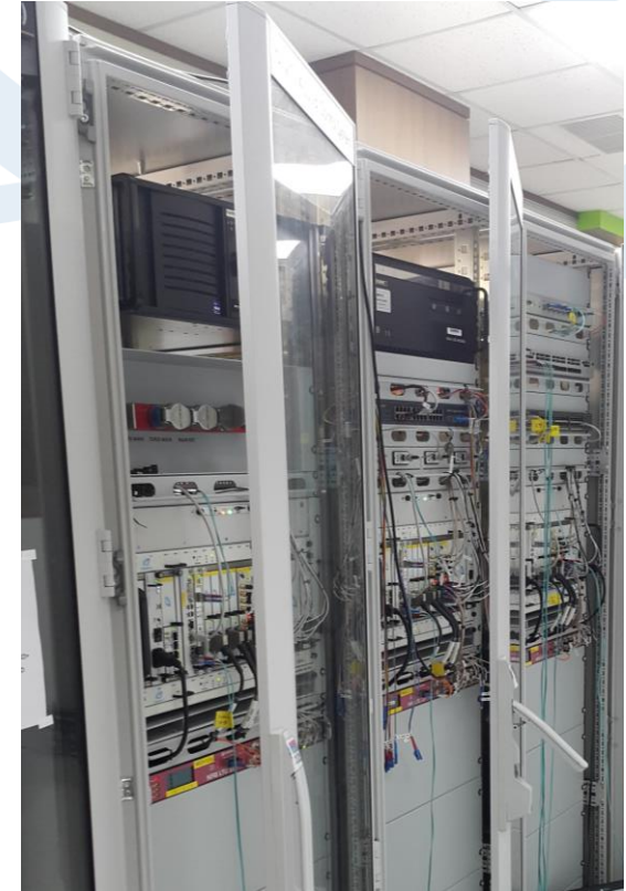
MTCA based loop controller of the plasma position via allocation of the power to the Superconducting Magnet
