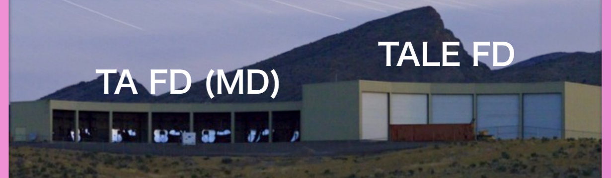
Middle Drum station
