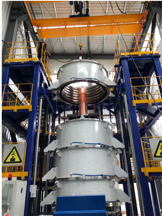
Into baking furnace on Oct. 28, 2019
