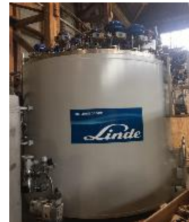
Helium recirculating tanks 2.5KW@4.5K cold box
